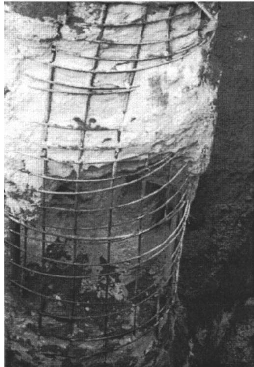
Fig. 1. Typical defect in bored pile constructed with polymer slurry
